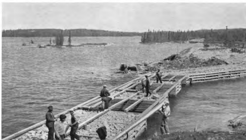
Indian workmen levelling up dam at Rocky Falls.
